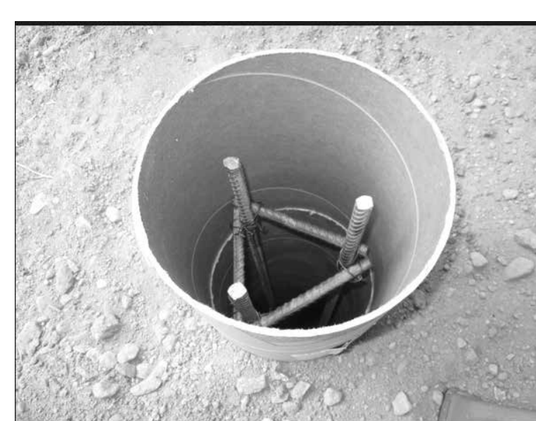
6 SONO TUBE - BEAM POST CONNECTION - LEDGER BOARD DETAIL NTS
