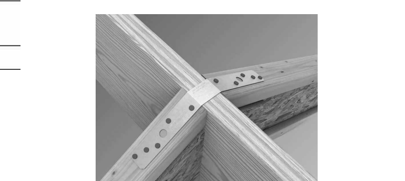
5 LSTA 1-1/4 in. x 12 in. 20-Gauge Galvanized Strap Tie NTS
